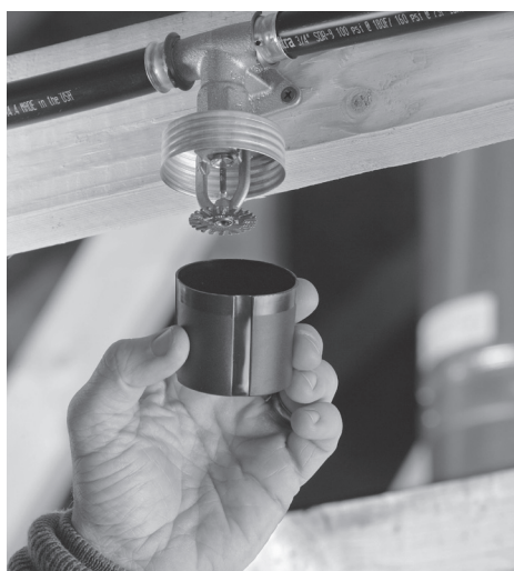
Keep heads within protective shell during installation
